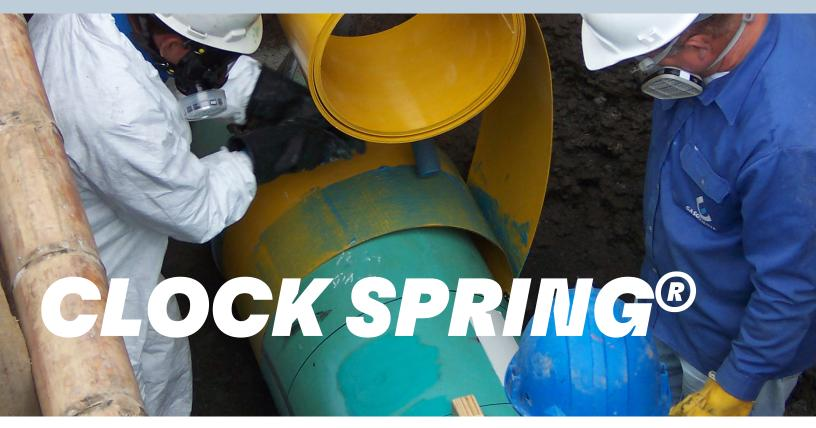
The Clock Spring composite repair sleeve and reinforcement system is uniquely designed for high pressure transmission pipelines. Made up of a pretensioned and pre-cured unidirectional e-glass composite coil, a high-modulus filler material, and a high lap-shear strength methyl methacrylate adhesive, it is proven to 8000 psi burst pressure, has a design life of beyond 50 years, and an installation history of more than 30 years, qualifying it as the first permanent repair in the industry.
