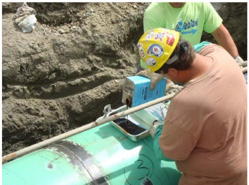
Figure 5: Preheat the pipe and apply primer (Section 4.1, 4.2)
