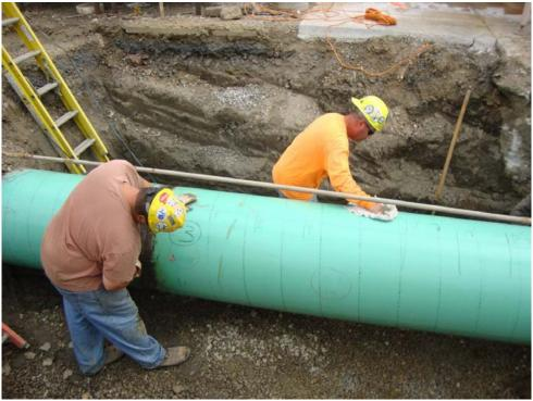
Figure 3: Cleaning the Surface (Section 3.2)
