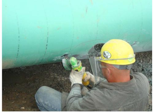
Figure 1: Remove all loose in disbonded coating (Section 3.1)
