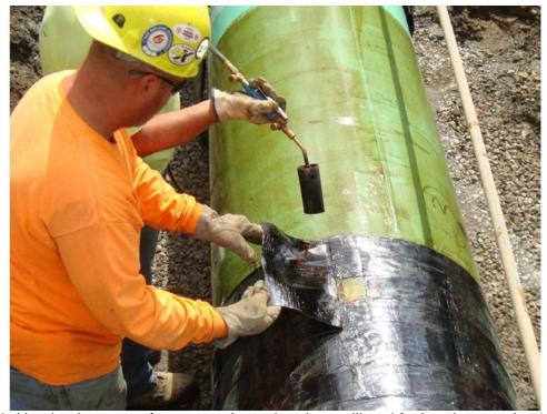
Figure 8: Heating last part of a precut piece, the piece will end facing down at the 1 o'clock position (Section 4.4)
