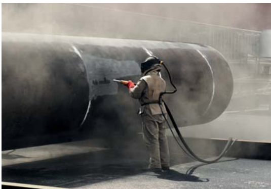
Conventional grit blasting
