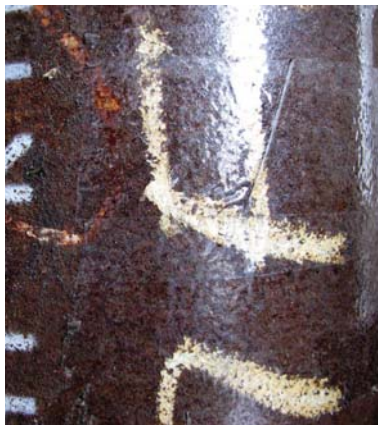
API 5L Piping
