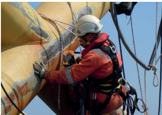
Bristle blaster® on an offshore platform
