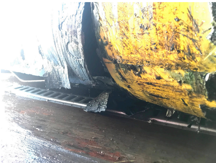
Figure 2. The repaired pipeline section was pressurised to and then held at that pressure for five minutes. After successfully holding the repaired pipeline section at the target value of 1455 psi (100.3 bar) for five minutes, pressure was increased until the pipeline finally ruptured at 2180 psi (150.3 bar). Interestingly, the rupture was not on the Clock Spring repair but on a section of pipe outside of the repair area. (Photo courtesy of CSNRI).
