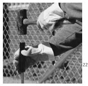
**ANSWER:** Time savings is achieved when using a driving sleeve or ERICO ground rod driver. If using a threaded rod, use the screw coupling and drive stud when driving the rod. For a plain rod, either steel or copperbonded, use the CADWELD driving sleeve listed below.
