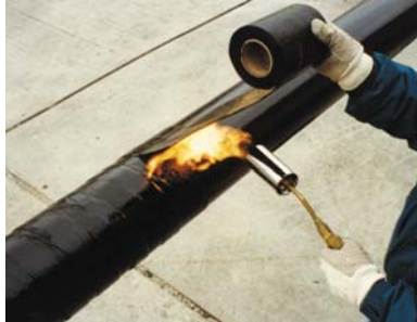
Pipeline rehabilitation and repair.
