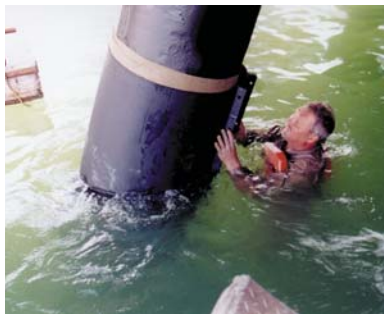
Low cost rehabilitation.
