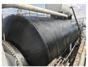
The flexibility and low profile of the DiamondWrap composite system allows installation even in areas with limited clearance.
