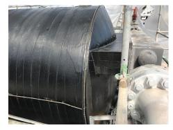
DiamondWrap can be installed on tees, elbows, and varied geometry without compromising the integrity of the repair. (Photo courtesy of ClockSpring|NRI)
