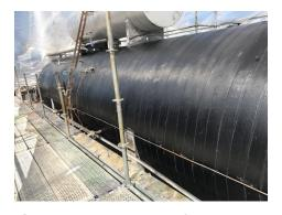
The composite system forms a pipe around a pipe, and each successive wrap increases the pressure rating, creating a finished repair that is stronger than steel. (Photo courtesy of ClockSpring|NRI)
