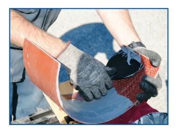
2) Trowel epoxy onto prepared substrate, and spread evenly with the included disposable putty knives. The putty knives will spread the epoxy more efficiently and easily over entire inside surface of FRP material. See table for approximate usage rates.
