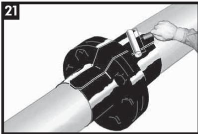
Apply a final rolling to secure the closure seal.
