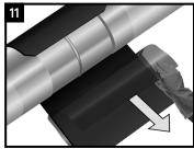
Centre the sleeve over the joint so that the sleeve overlaps between the 10 and 2 o'clock positions. Press the underlap firmly into place and remove the remaining release liner.
