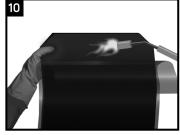
Partially remove the release liner and gently heat the underlap approximately 150mm (6") from the edge. Sleeve temperature shall be at least 18°C (65°F) at time of installation.
