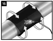
Continue heating from the centre toward one end of the sleeve until recovery is complete. In a similar manner, heat and shrink
