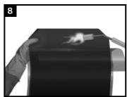
As an option, slightly trim corners of preattached closure. Partially remove the release liner and gently heat the underlap approximately 150 mm (6") from the edge.
