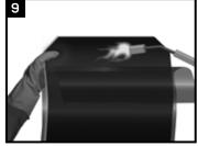
Partially remove the release liner and gently heat the underlap approximately 150 mm (6") from the edge.
