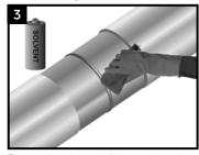
Ensure that the mainline coating edges are beveled to 30°. If there is the presence of oil, grease, or other surface contaminants; clean the exposed steel and adjacent pipe coating with a solvent cleanser.
