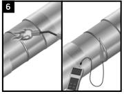
Pre-heat the joint area to the minimum of  $65^{\circ}$ C ( $150^{\circ}$ F). Using a temperature measuring device, ensure that the correct temperature is reached on the steel and at least 50mm (2") on each side of the sleeve.
