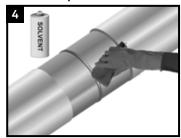
Ensure that the PE coating edges are beveled to 30°. Clean exposed steel and adjacent pipe coating with a solvent cleanser to remove the presence of oil, grease, and other contaminants.
