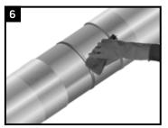
Wipe clean or air blast the steel and pipe coating to remove foreign contaminants.
