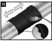
Shrinking has been completed when the adhesive begins to ooze at the sleeve edges all around the circumference. Finish shrinking the sleeve with long horizontal strokes over the entire surface to ensure a uniform bond.
