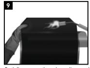
Partially remove the release liner and gently heat the underlap approximately 150 mm (6") from the edge.
