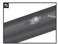
Preheat the area with a low to moderate intensity flame to substantially cure the epoxy and warm the surface. Skip to box 10
