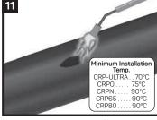
Warm the damaged area (repair zone + 50mm (2") overlap) to remove moisture and assist in adhesion.
