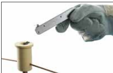
Fig. 15 Aiming the flint igniter from the side, ignite the starting material on the mold cover. Withdraw the igniter quickly to prevent fouling. Allow approximately 30 seconds for completion of the reaction and solidification of the molten material.
