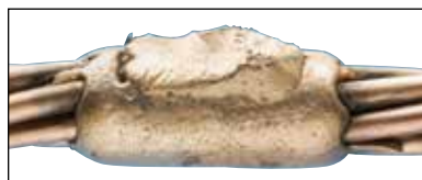
Fig. 29 Completed Cadweld connection.
