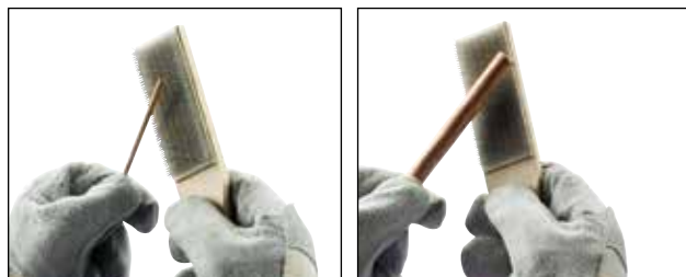
Fig. 5 Next, use a wire brush to further prepare the surface of the conductors and ground rod (Cadweld T-313 or T-314 brush). Scrape the outer surface to remove dirt and oxidation. You will notice a slight color change.
