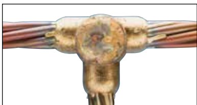
Fig. 26 Completed Cadweld connection.
