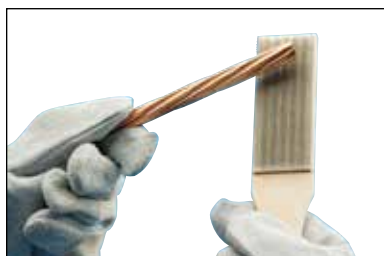
Fig. 12 Next, use a wire brush to further prepare the surface of the conductors (nVent ERICO T-313 or T-314 brush). Scrape the outer surface to remove dirt and oxidation. You will notice a slight color change.
