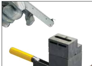
Fig. 24 Aiming the flint igniter from the side, ignite the starting material on the mold cover. Withdraw the igniter quickly to prevent fouling. Allow approximately 30 seconds for completion of the reaction and solidification of the molten material.
