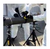
Slide the center of the stopper "sphere" onto the center of the leak and apply pressure to maintain the position of the Leak Stopper™ while its tightened.
