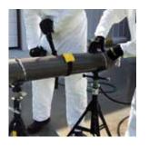
Being mindful of the pinch points along the edges of the stopper, use the rachet to tighten the band, resetting the metal bracket onto the teeth and closing the rachet until no more pressure can be applied, and the leak has stopped.
