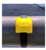
Use the back of the tool to trim the excess slack from the band and provide a smooth profile across the pipe.
